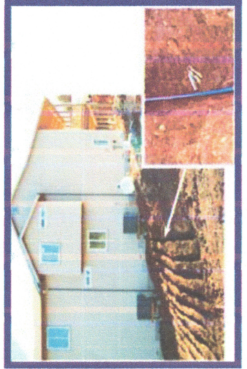
Typical Drip Installation
